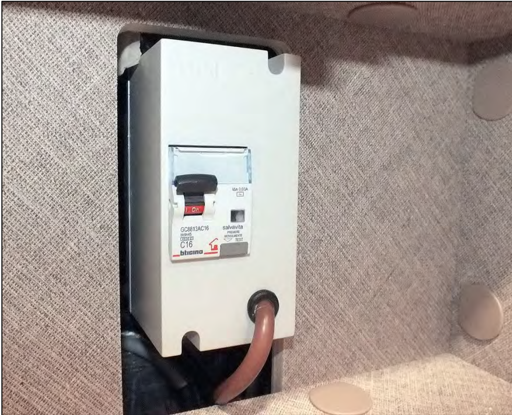
230 V fuse with RCD (sample illustration)
