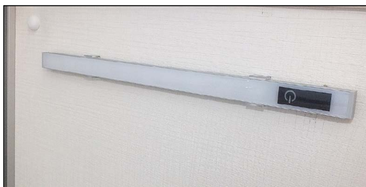
Wall lighting strip, with sensor button
